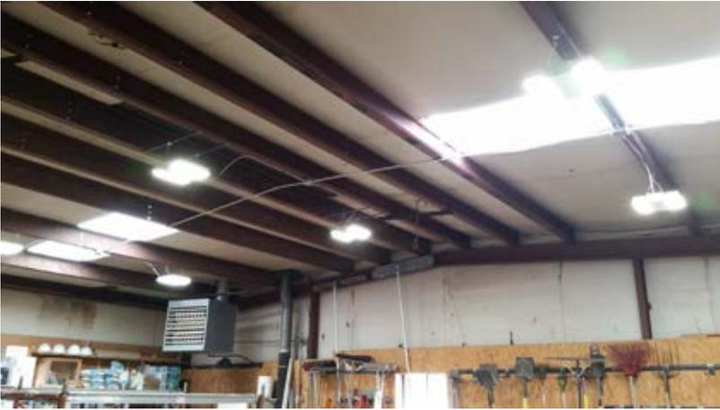
The Park's Department shop received a complete relighting of the shop area. This consisted of removing old 8ft fluorescent lights and piping and installing new LED lights and energy metallic tubing (EMT). The switching
